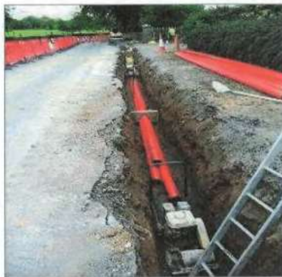
Figure 2 - Typical 38kV Underground Duct Installation
